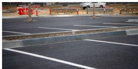
Figure 1. Waste tyre permeable kerb and channel system
