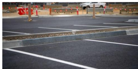
Figure 1. Waste tyre permeable kerb and channel system
